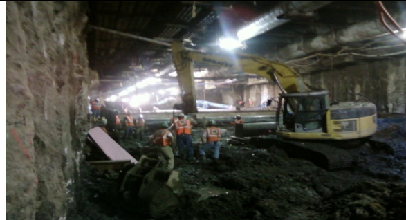
Work in progress under decking
