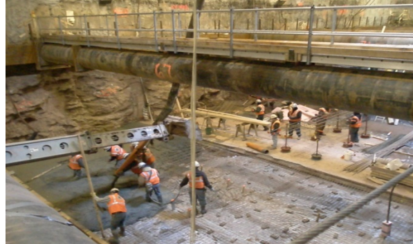
Placement of concrete mud mat
